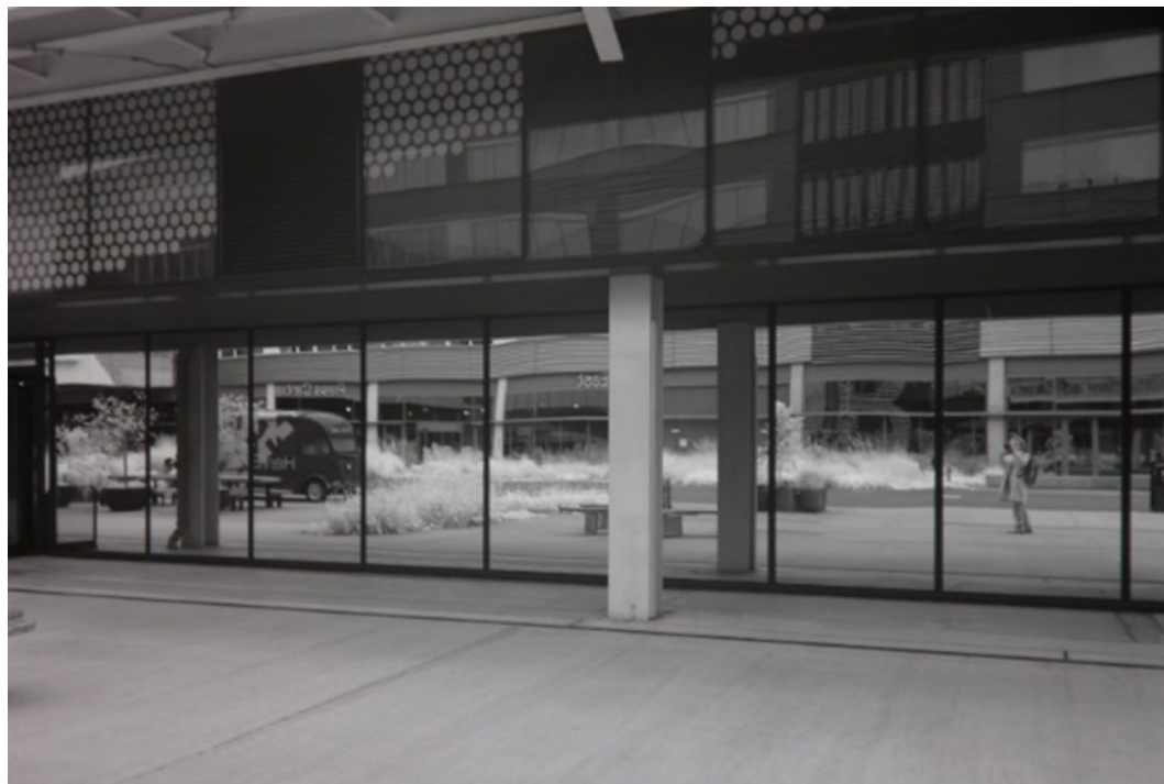
Fig. 1. Infrared photograph of the front of the Here East building (~ 800–1000 nm). The glazing reflects infrared light away, resulting in the mirror-like appearance of the windows. The photographer (EB) can be seen on right hand side of the reflection.
