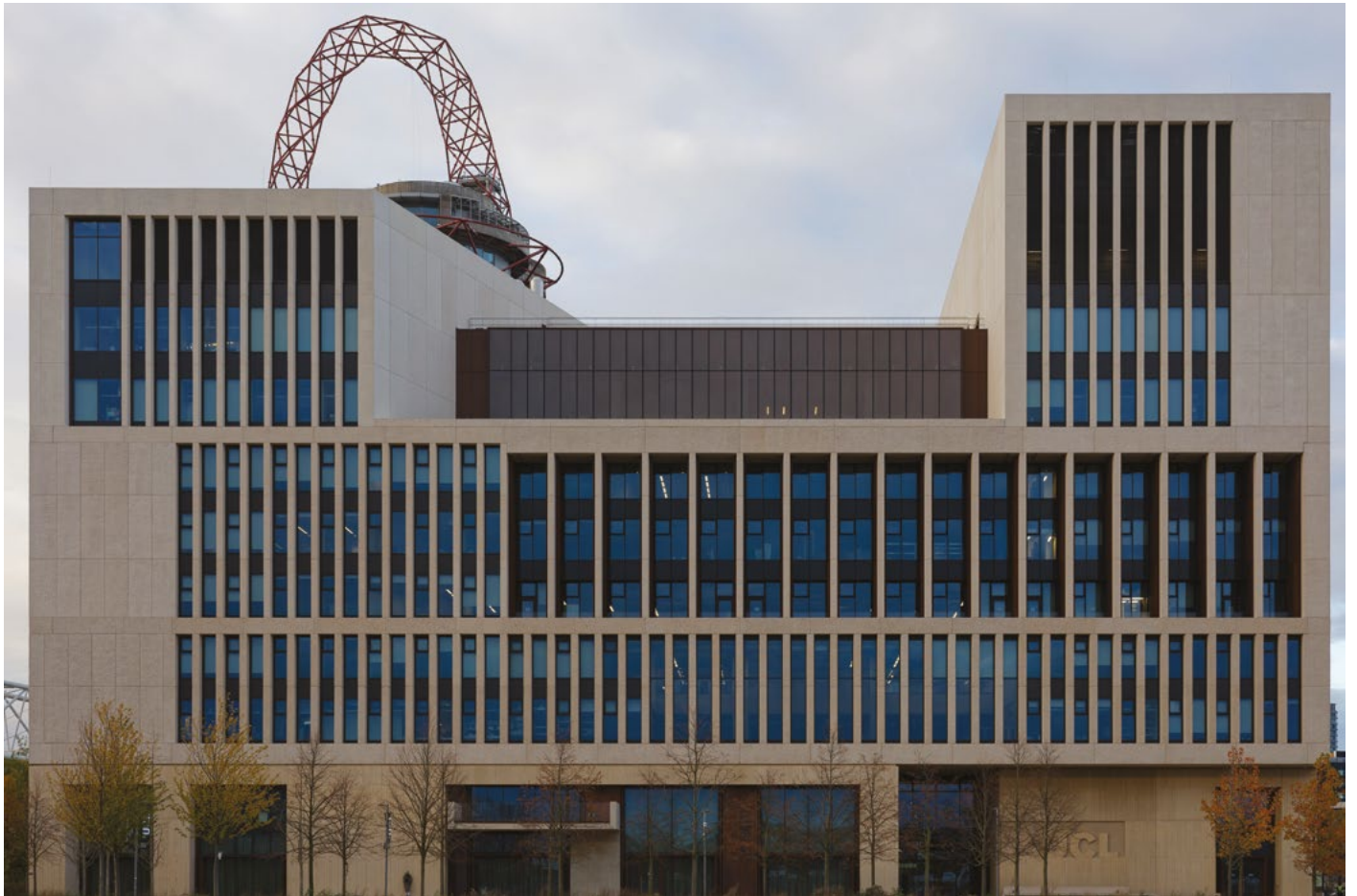
UCL East Marshgate building at Stratford Waterfront Campus is the largest single building at UCL, and part of the largest expansion of the university since it was founded almost two hundred years ago (image credit: Edward Barrett).
